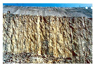
Figure 1: Example of controlled blasting rock face.
