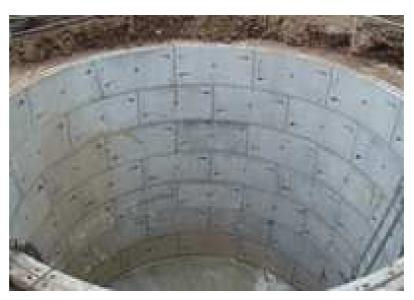
Figure 2: Example of segmental lining for shaft sinking (perco.co.uk).
